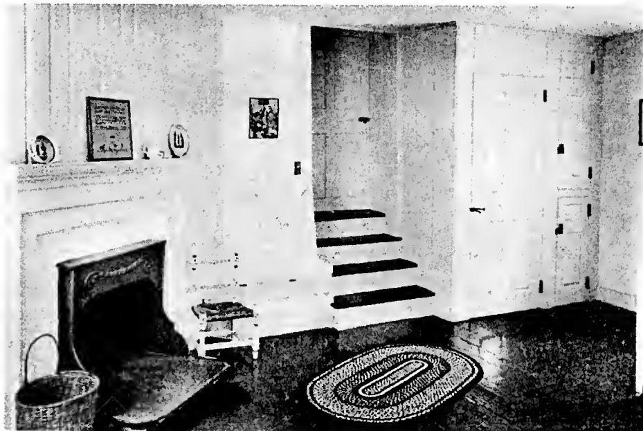
Figure 40 Second Floor South Room, Center Section of Main House, 1925
